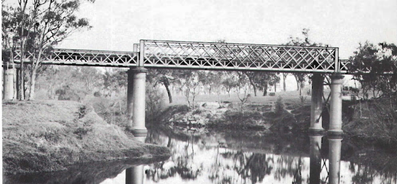
An early photograph of the old railway bridge at Heyington. Cast iron piers support the lattice girders of the river span and the two side spans. Timber structures formed the approaches.
